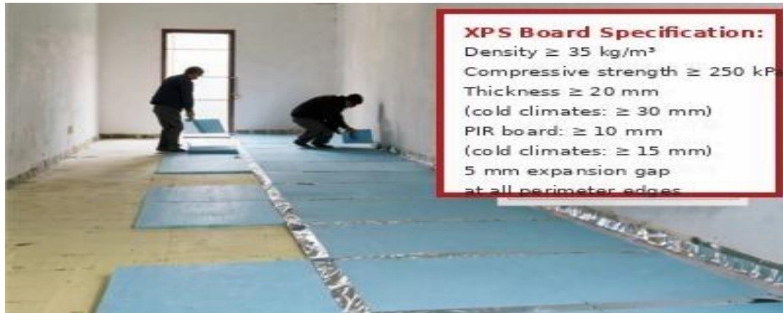
XPS insulation boards being laid; foil tape sealing joints
