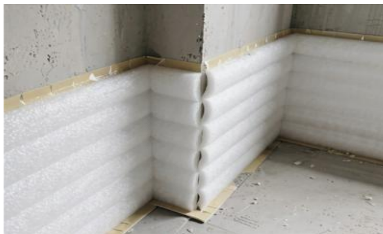
EPE perimeter insulation strip installed at wall/floor junction, corners mitre-cut at 45°
