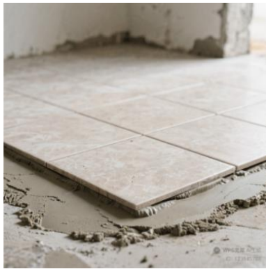
Cement mortar + floor tiles
