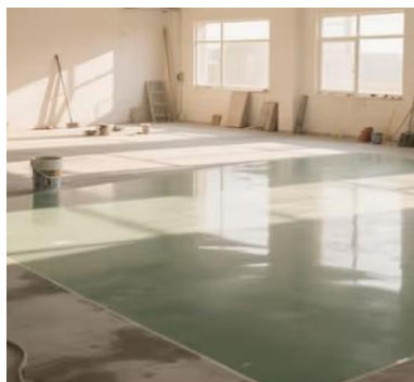
Cement mortar plus epoxy flooring
